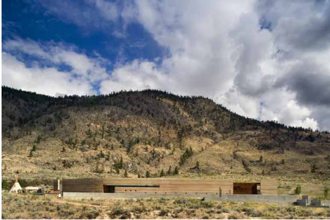
Photo of Nk'Mip Desert Cultural Centre, Osoyoos Indian Band. Retrieved from https://nkmipdesert.com/our-sustainable-building/
