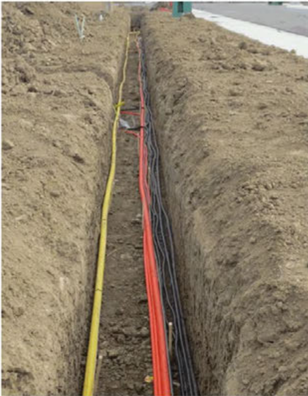
Shallow Utility Installations in Residential Subdivisions
