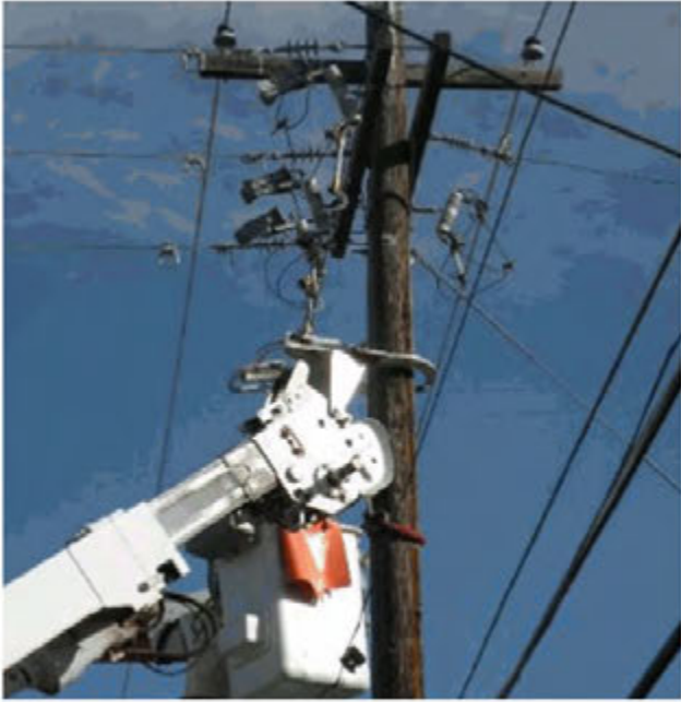
Overhead Main Line Assessment
