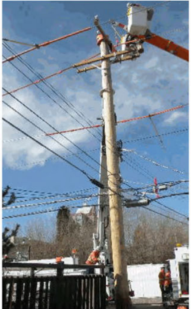
New Overhead Main Line Brought into Place
