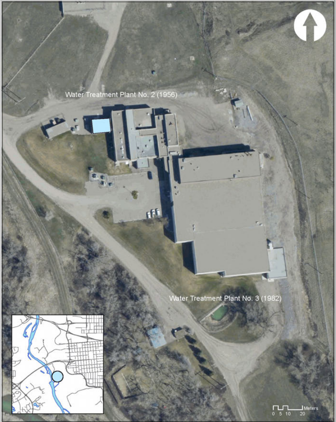
Water Treatment Plant No. 2 HLP Switchgear Upgrade
