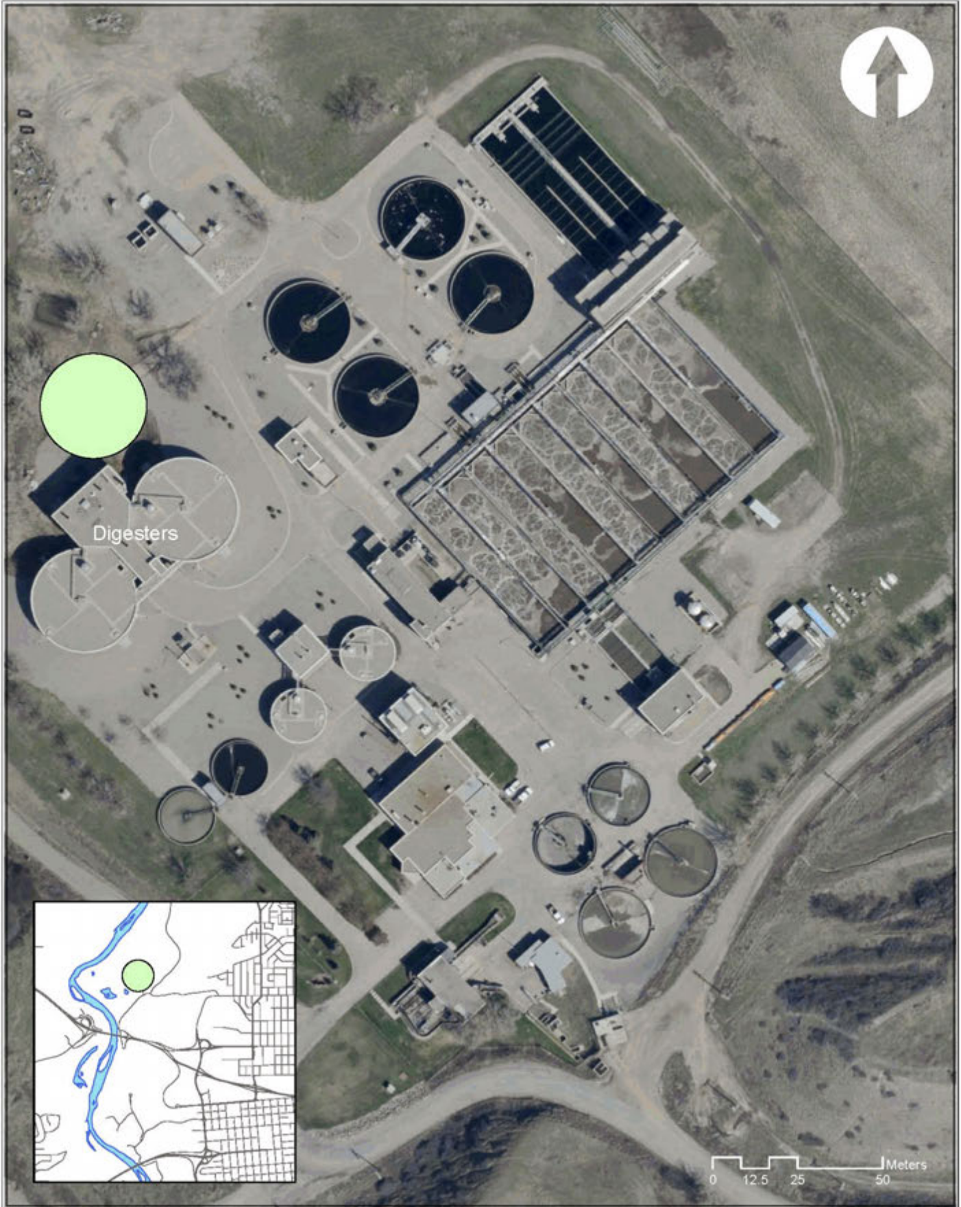
Wastewater Treatment Plant Additional Digester
