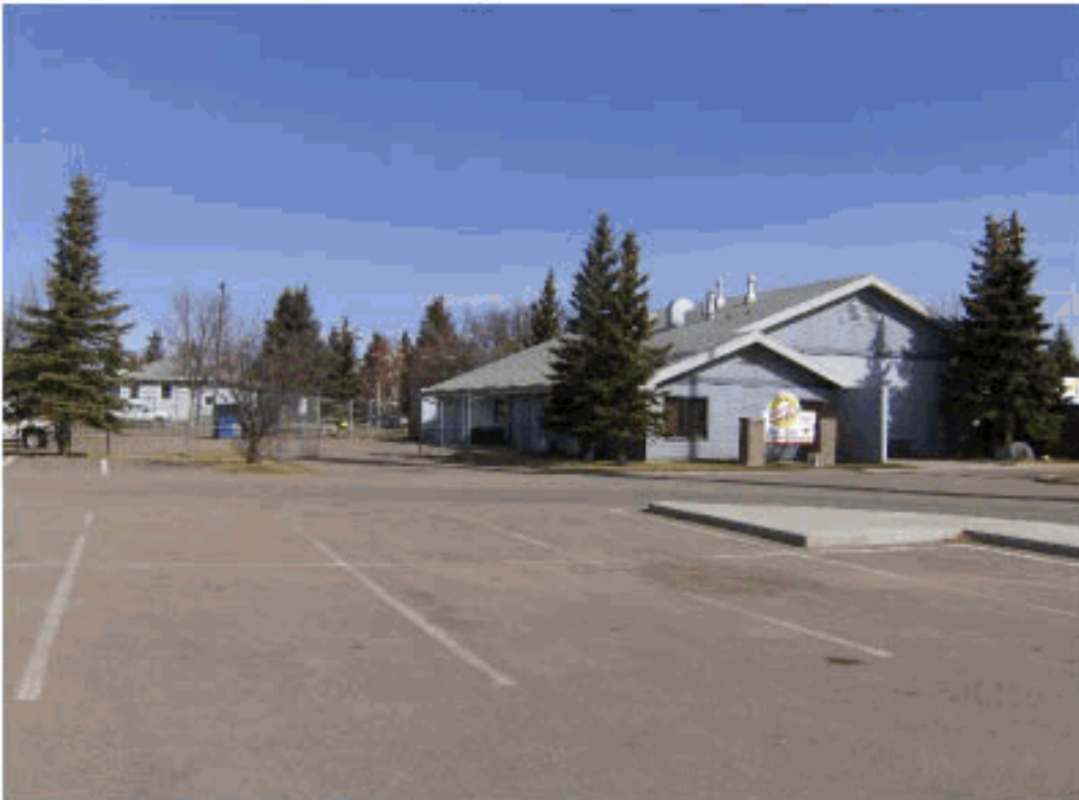
Former Parks Depot in Henderson Lake Park
