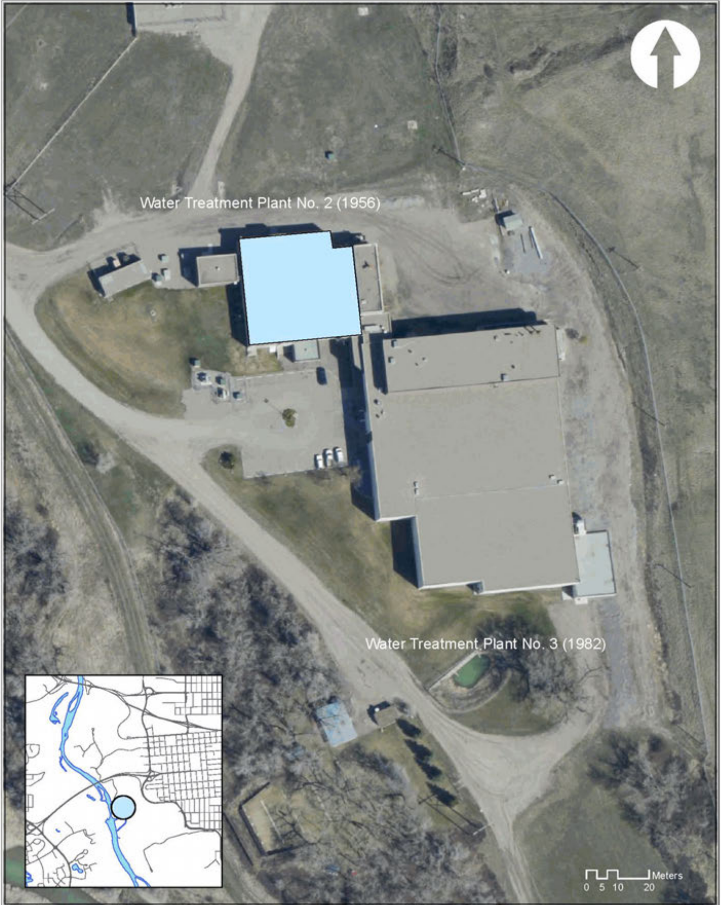
Water Treatment Plant Process Redundancy
