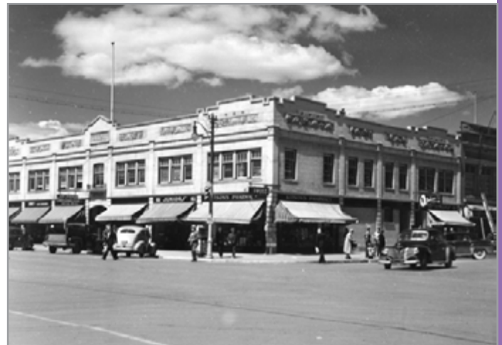
McFarland Building, corner of 6th Street & 4th Avenue (1948)
