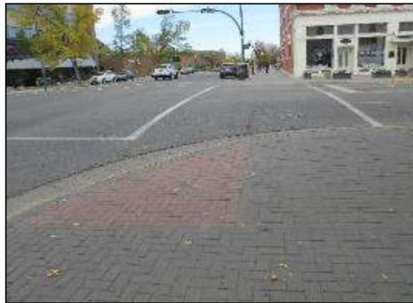
Figure 6-27: Example of a Blended Curb Ramp
