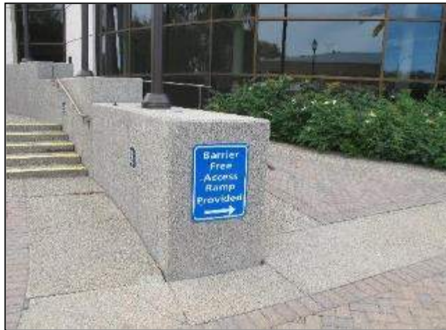
Figure 6-19: Example of Barrier-Free Access Ramp
