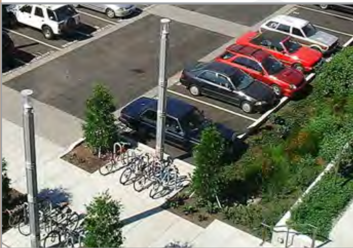
Surface runoff from parking is treated by vegetated system
