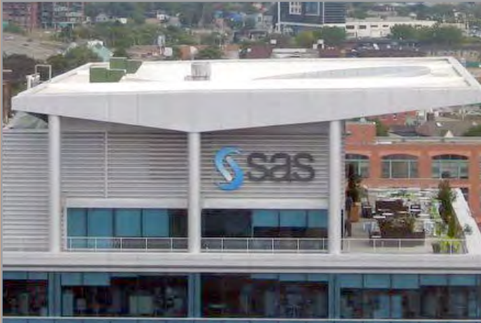
This roof captures rainwater for use in building toilets
