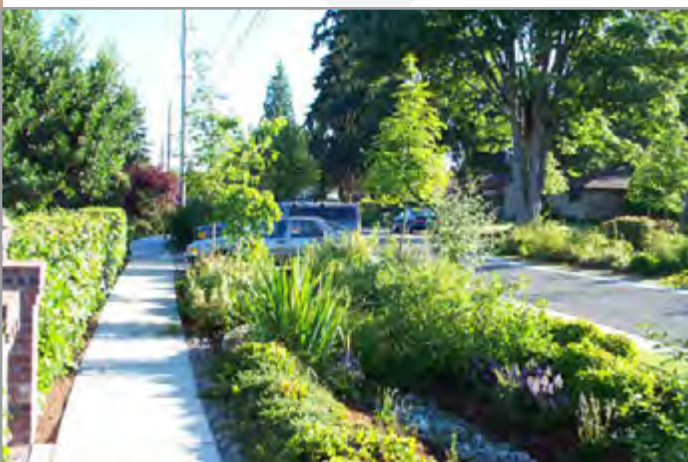
Surface runoff from the street is captured in a naturalized swale
