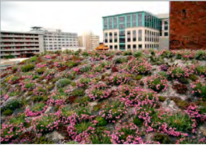
Green roofs reduce urban heat island effects and have insulating properties
