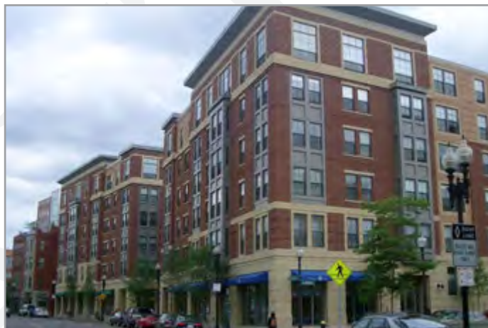
Material variety used to articulate the building: stone base, brick facade and a variety of details to articulate the base, middle and top
