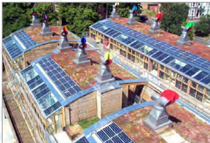
Green roofs, natural ventilation and solar panels
