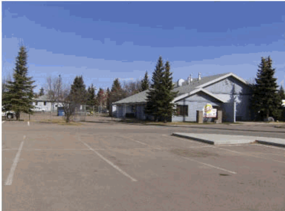
Former Parks Depot in Henderson Lake Park
