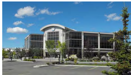
A health-sciences firm that is part of an office park in a business industrial area
