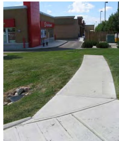
Sidewalk to nowhere... An example, from a retail development, of a public sidewalk that is not continued onto private lands. This does not promote pedestrian connectivity
