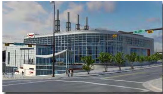
Enmax's Downtown Calgary District Energy Centre Source: Enmax Corporation "www.enmax.com"
