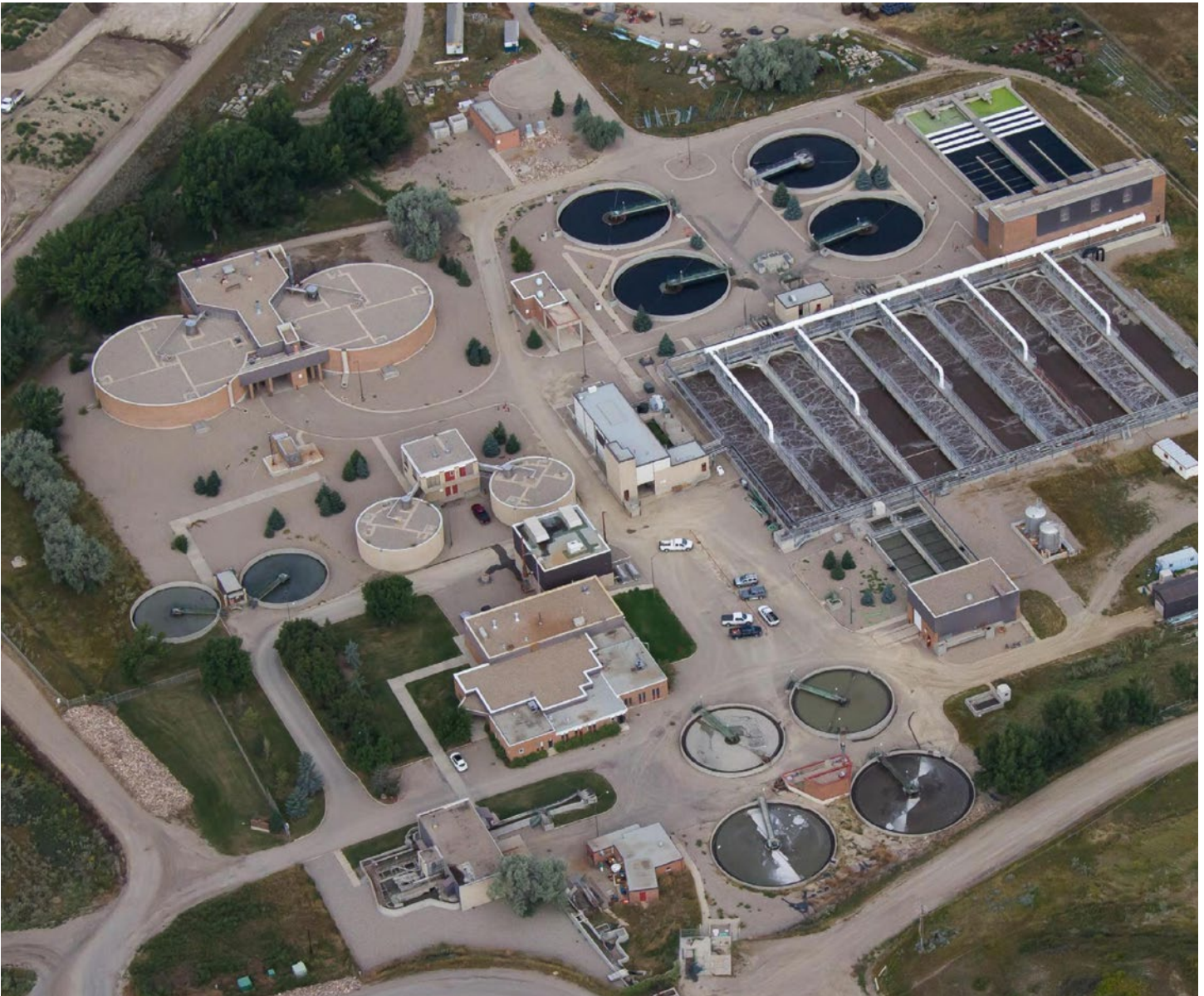
Wastewater Treatment Plant
