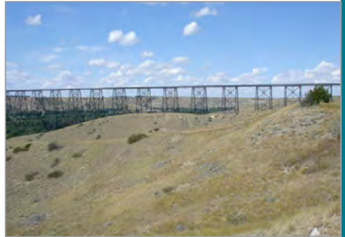
The High Level Bridge
