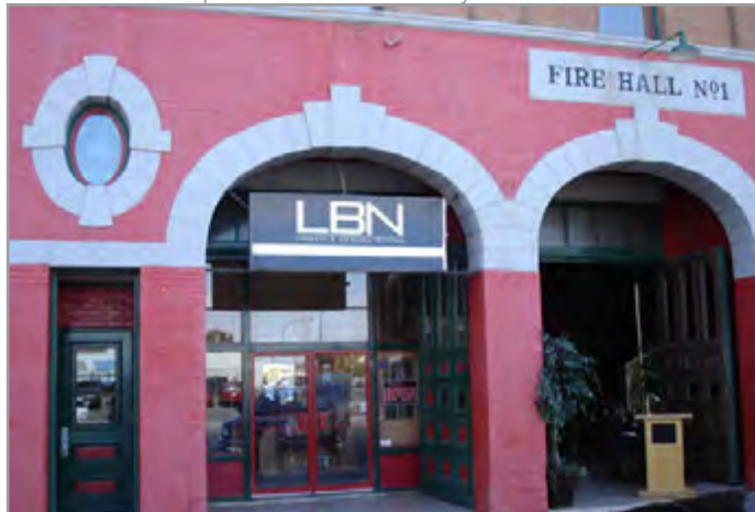
Adaptive re-use of heritage buildings
