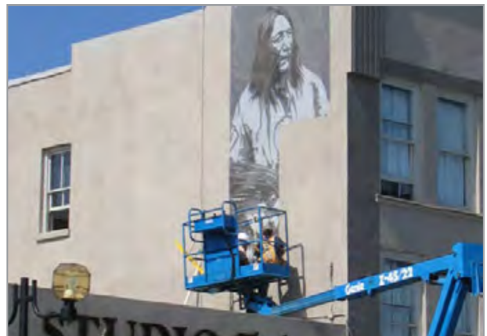
Heart of Our City Campaign: Installation of Murals
