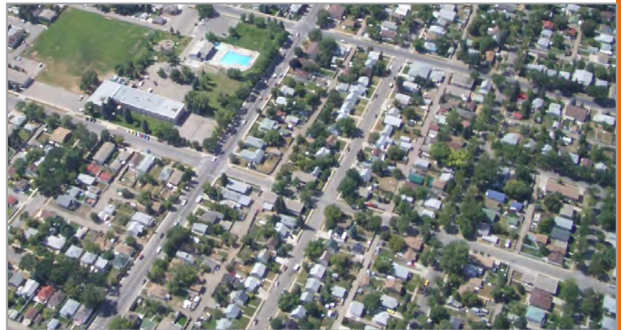
2. The traditional gridiron street and block pattern in Lethbridge is designed for walking
