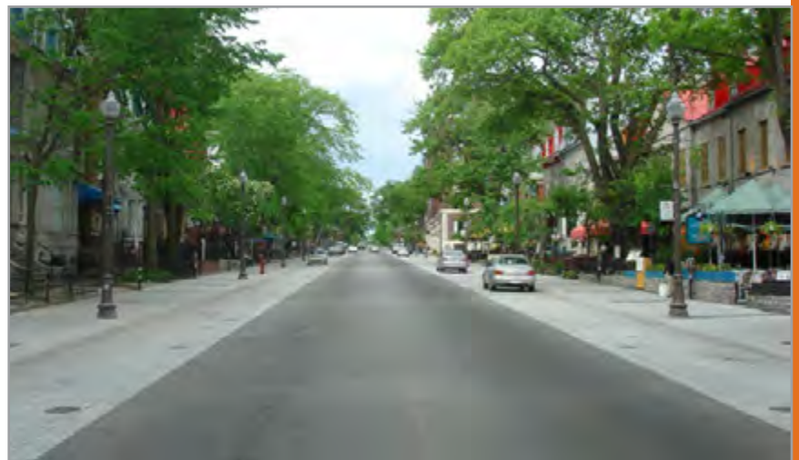
8. Special paving for on-street parking lanes to visually minimize width of roadway
