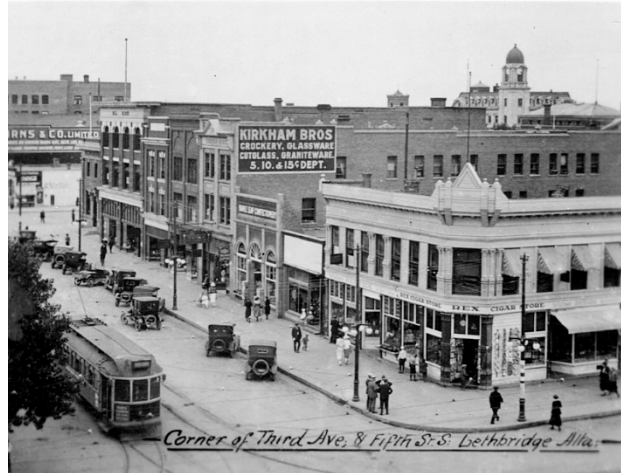
Figure 41: Corner of 3 rd Avenue and 5 th Street South. (Source: Galt Museum & Archives)
